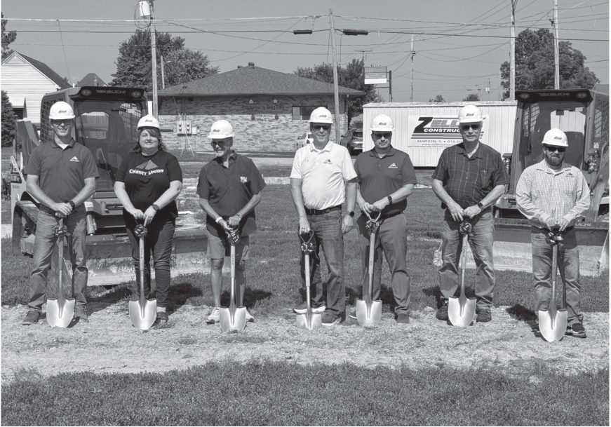
Groundbreaking for our new Marion location at 105 West DeYoung Street on July 11, 2025.
